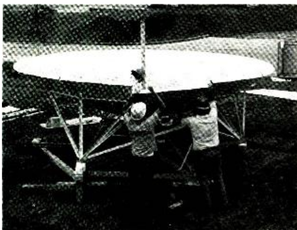
The dish is constructed atop the base
